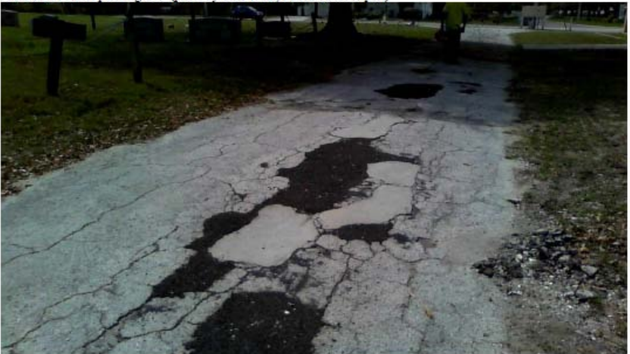
Photo RPS Pothole patching CW (photo by Cliff Work, March Status Report)
