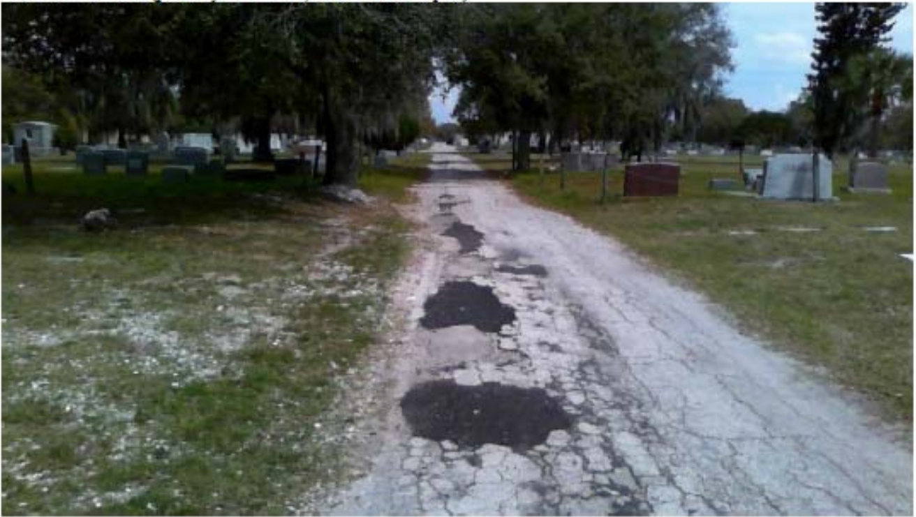
Photo RPS Pothole patching CW (photo by Cliff Work, March Status Report)
