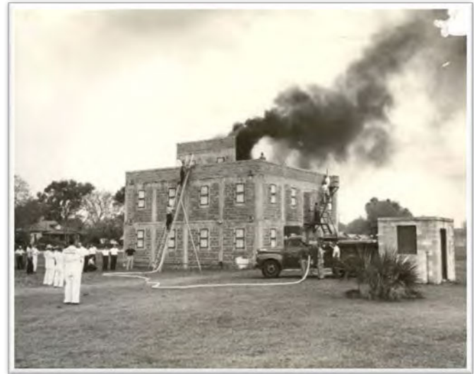
Burn building at original campus
